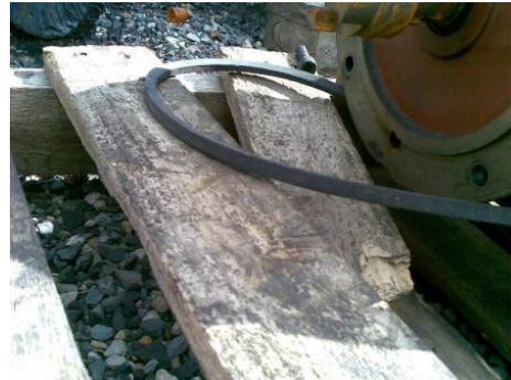
X Broken planks
